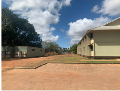
1 CARPARK VIEW TO EXISTING MOTEL
