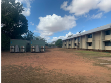
2 CARPARK VIEW TO EXISTING MOTEL
