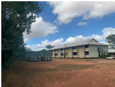
3 CARPARK VIEW TO EXISTING MOTEL
