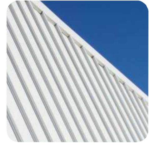
#05 ROOF / WALL SHEETING FINISH AND APPLICATION OF ROOF / WALL CLADDING
