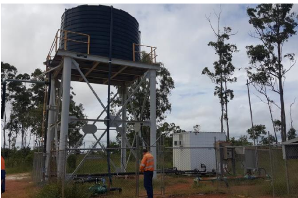
Figure 3-13 Elevated Storage Tank
