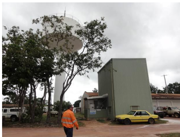
Figure 3-4 Elevated Water Storage
