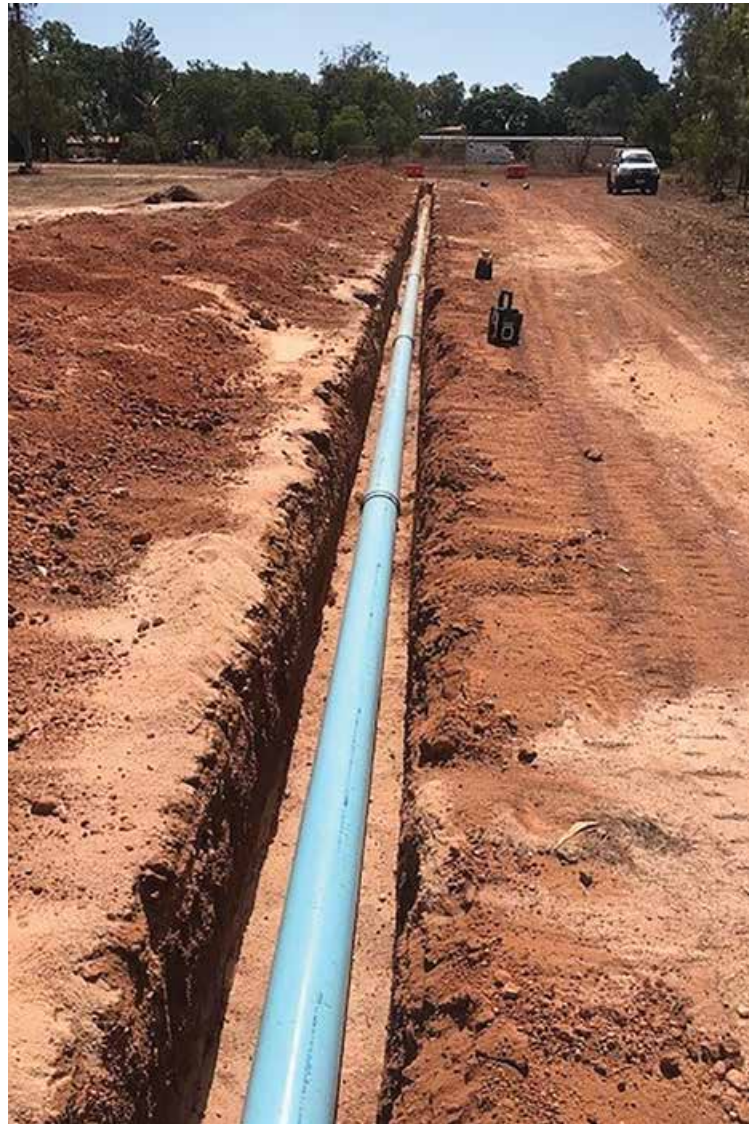
Trunding water main upgrade
