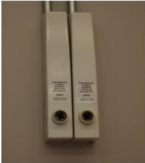
Photograph: Close upper level louvers with winders
