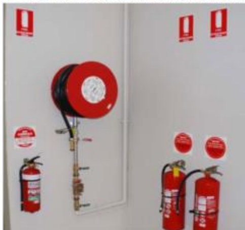
Photograph: Open green valves on fire hose reels
